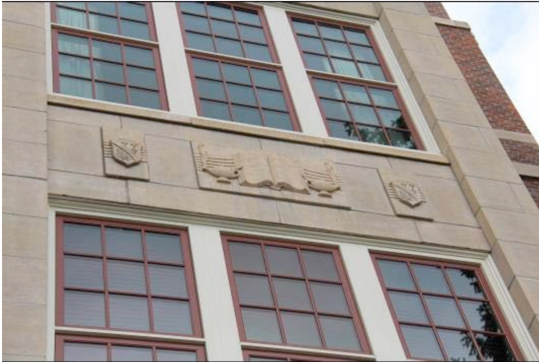
0010 Detail photo of cultured stone panels and raised inserts above the front entry. View to north.
