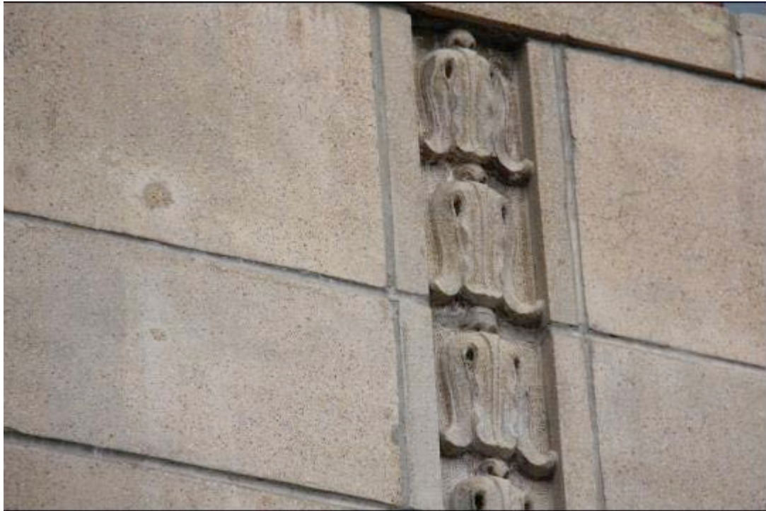
0011 Detail photo of cultured stone panels and lotiforms that are distributed around the building.
