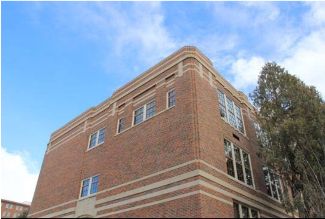
0006 Photo looking up at the architectural detail on the southwest corner of the building.
