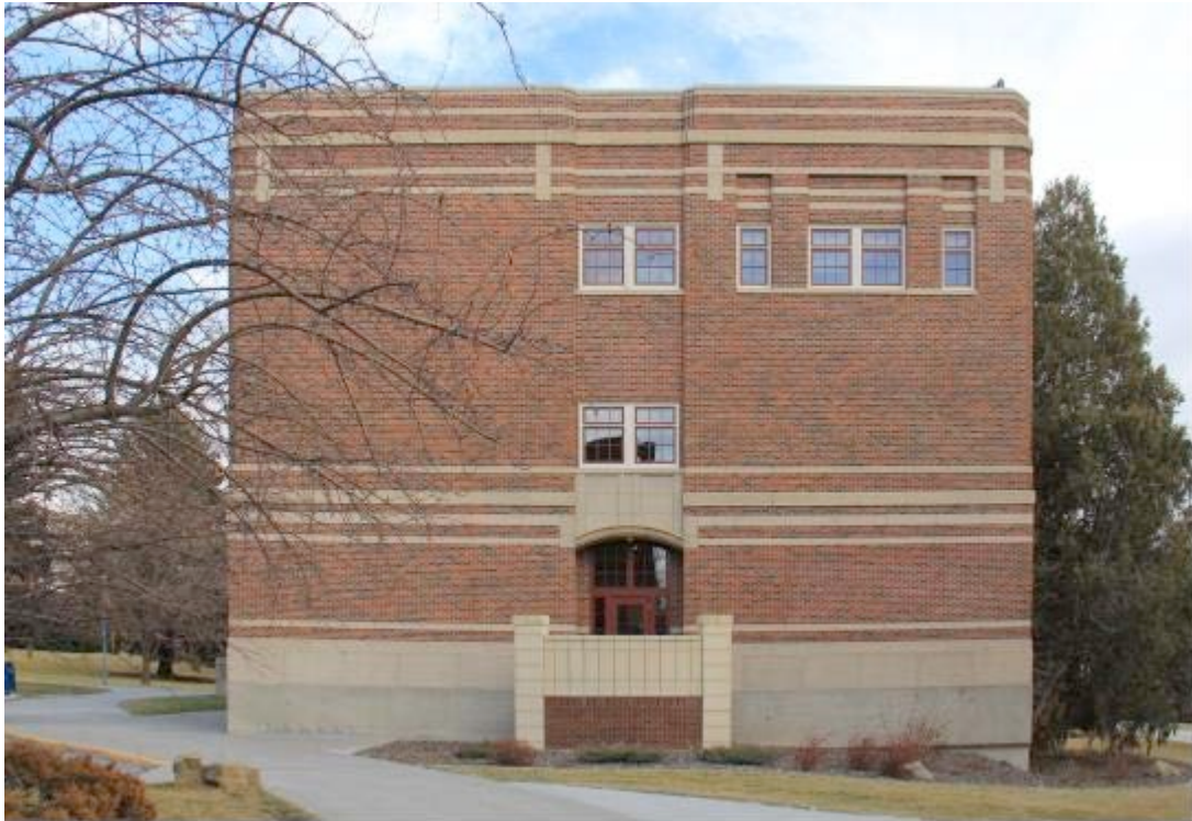
0003 Photo of the west side of McMullen Hall. View to east.
