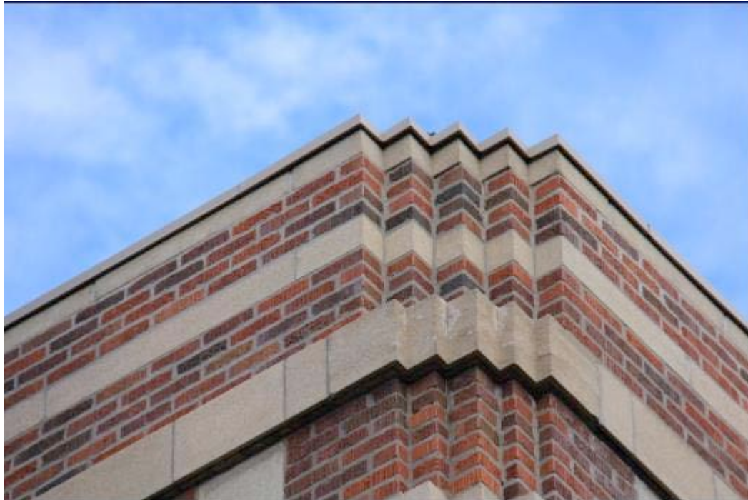
0007 Photo of the architectural corner detail on the southwest corner of the building. This is typical of all corners.
